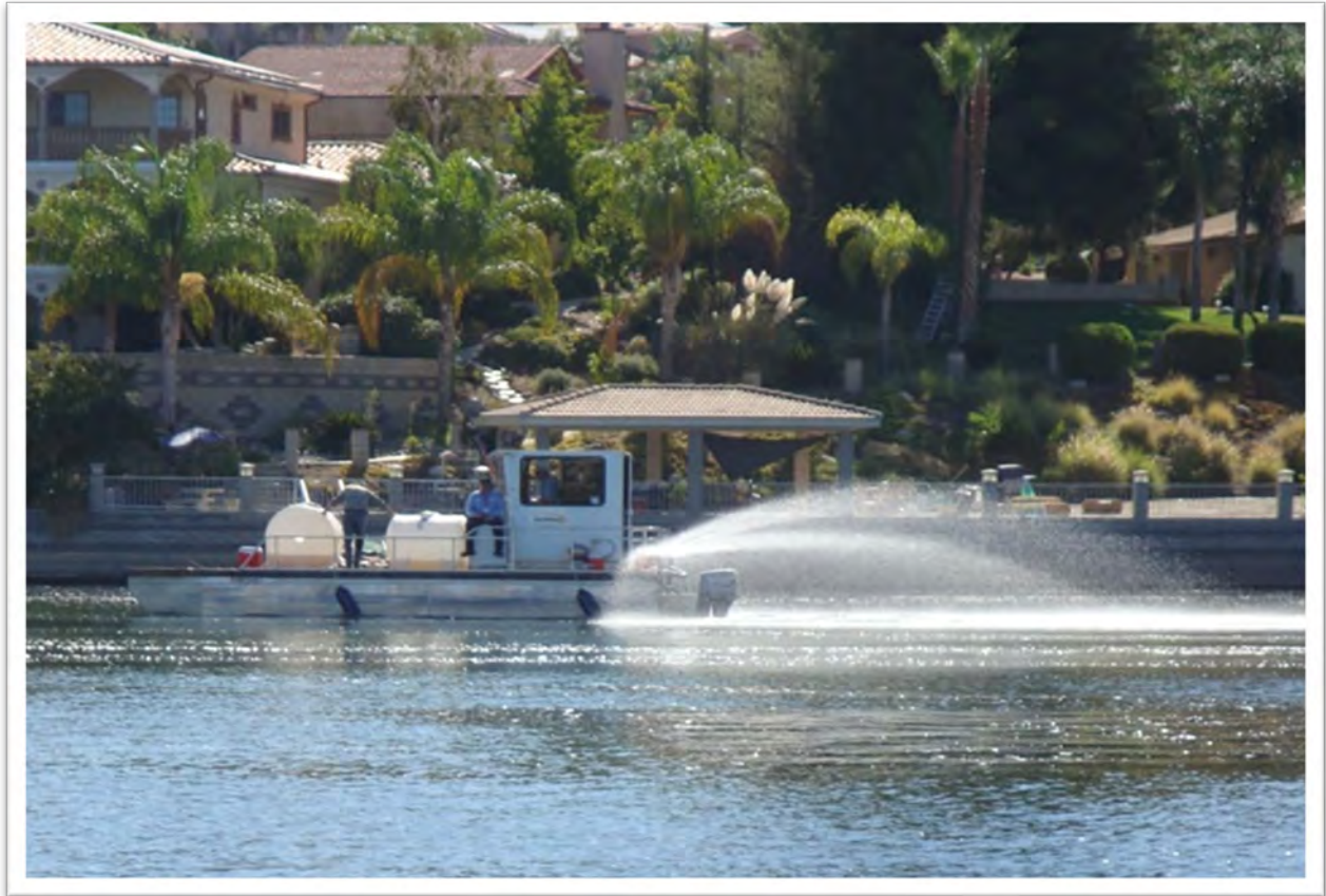
Aquatechnex biologists applying Alum on Canyon Lake
