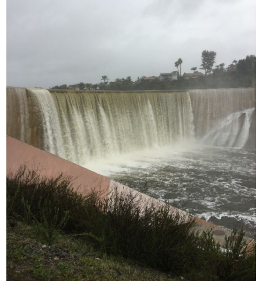
Storm Event Monitoring at Canyon Lake Spillway in February 2019
