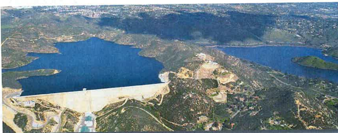
A pipeline between Olivenhain Reservoir (left) and Hodges Reservoir (right), can deliver water from Hodges into the Water Authority's aqueduct system.
